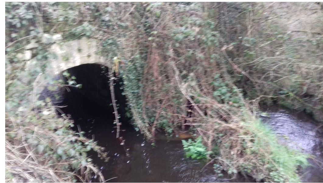
Photo No. 9 A
